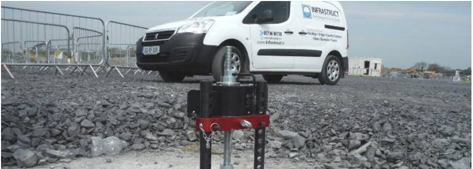
Proof Load Testing to 140kN
